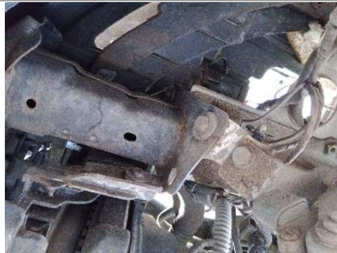
Main Beam Left
