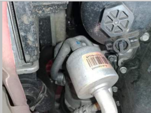
Air conditioner pipes
