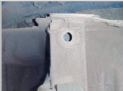
Main Beam Left
