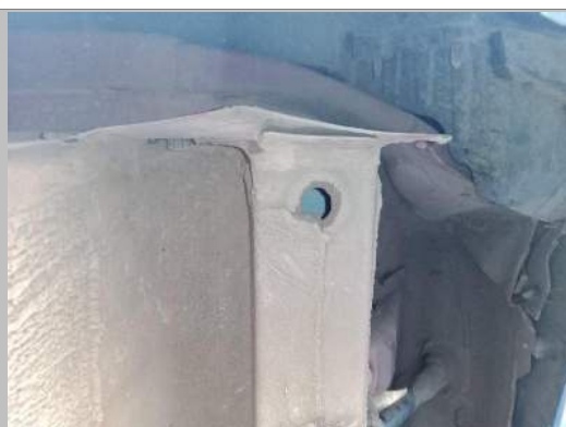
Main Beam Right
