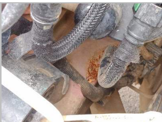
Main Beam Right
