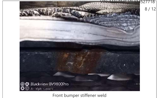
Front bumper stiffener weld
