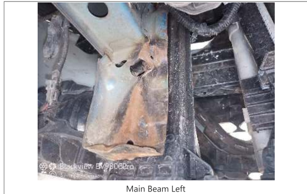
Main Beam Left
