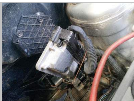
ECU is loose
